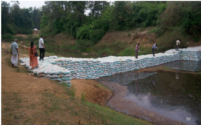
Photo : 15 (NREGA 2006-07) Construction of Bund at Kakkadavu, Vellamunda GP Mananthavady Block, Wayanad District
