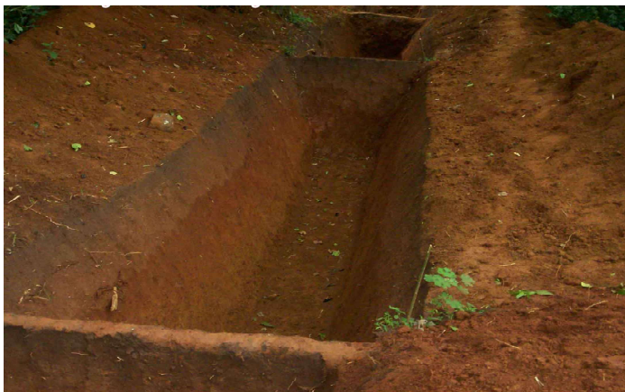
Photo : 17 Vellarody Colony Perculation Trunch Thirunelly GP, Mananthavady Block Waynad District
